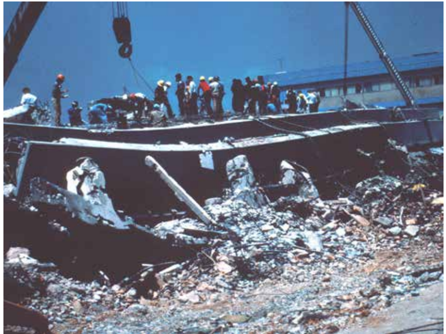
▲ Das eingestürzte General Hospital in Mexico City 1985
